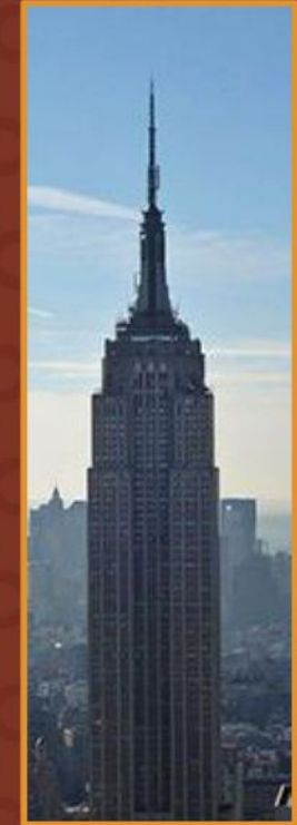
The Most Famous Structural Steel Structures in the World
