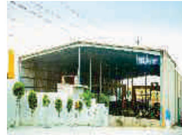
BCC PRECAST PLANT
